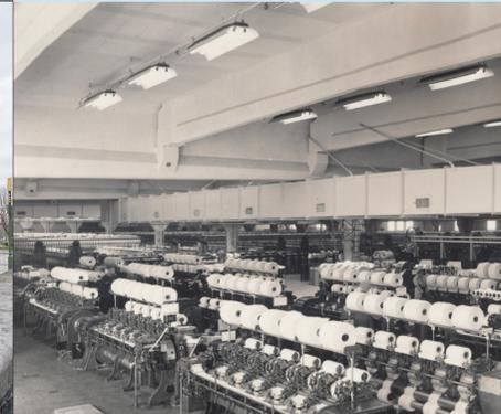
Factory hall with combing machines, preparation for spinning. Photograph Remy Bulters, ca. 1958-1970.
